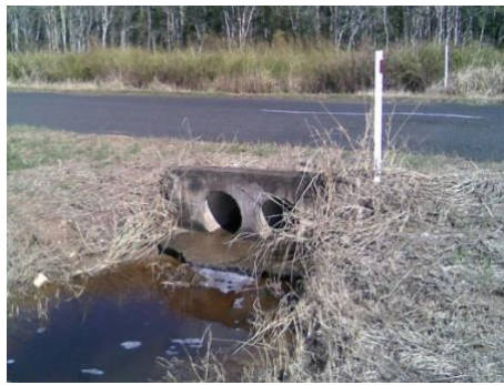
Road Cross Culvert
